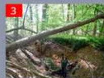
3 Southern Aster Boulevard Outfall - Before
