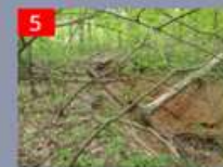
5 Southern Aster Boulevard Outfall - Before
