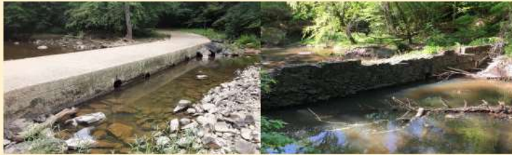
Figure 2 (left): the Concrete Bridge site. Figure 3 (right) the Billy Erwin Dam.
