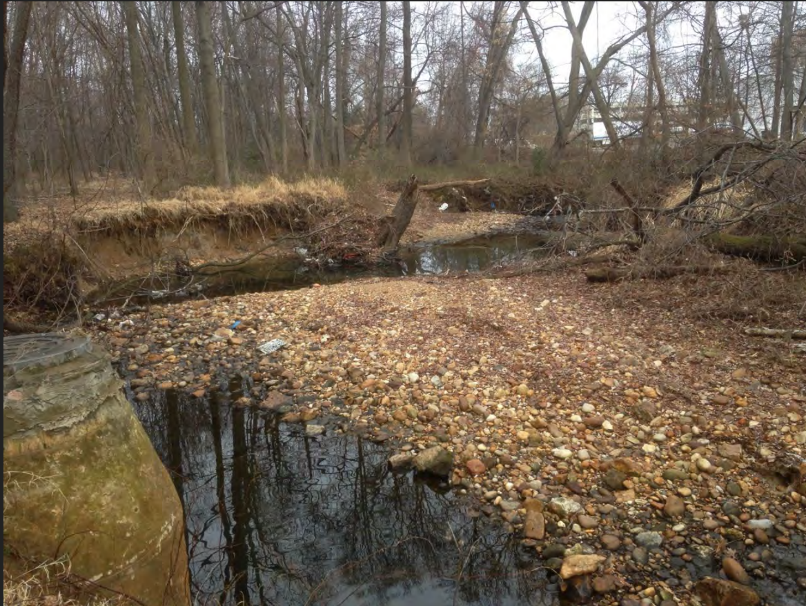
Pre-construction with exposed sanitary sewer manhole
