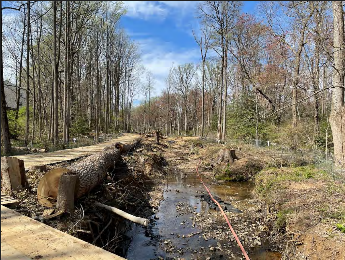
Cleared with construction access installed
