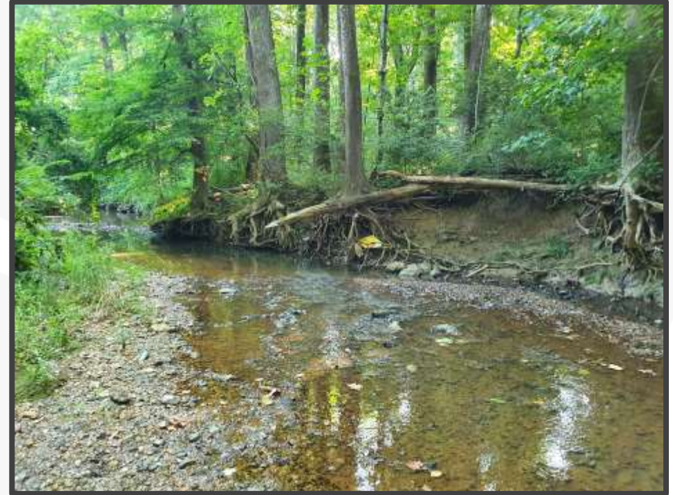
Representative Bank Erosion
